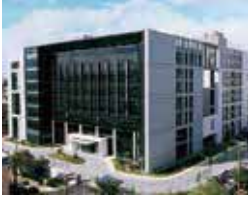
Taoyuan Technology Center (Green Building)
